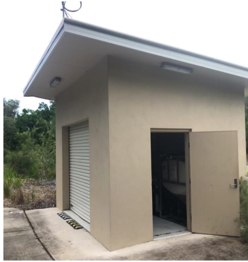
Figure 2 – Example of typical standards MHL Dosing building
