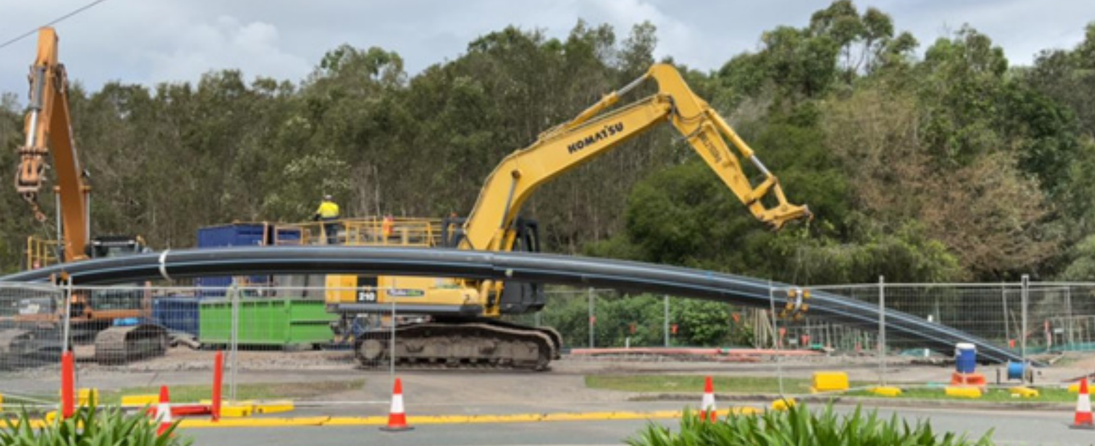
HDD pipe pullback Bellflower Rd
