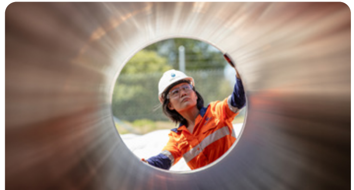
Program Engineer, Gwennie Lam, inspecting the pipes before they go underground.
