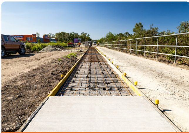
Reinstatement of shared user pathway along the Bells Creek Arterial (BCA).
