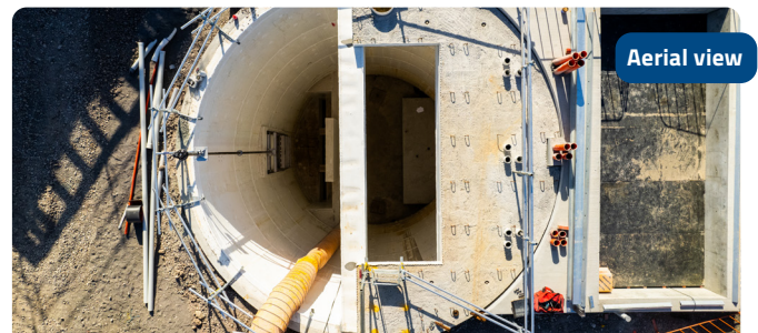
Aura Wastewater Project's 15 metre deep wet well at the new pump station.
